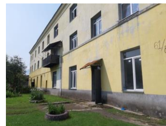
Drohobych, apartment building
